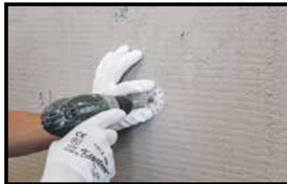
Verdübelung MIT MAPETHERM TILE FIX15
